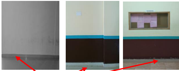
Figure 2: Wall image with skirting
